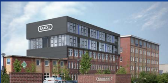
SAACKE Head office Bremen (Germany)
